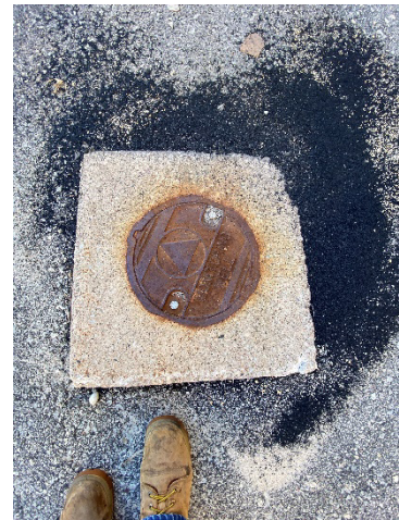
Monitoring well east side of school
