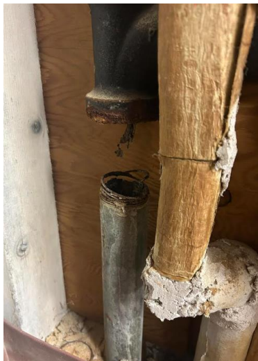
Old plumbing, rusted through pipes, disintegrating insulation, and damage caused by pipes that leaked or rusted through.
