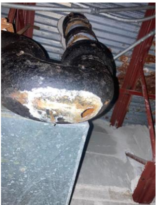
Old plumbing, rusted through pipes, disintegrating insulation, and damage caused by pipes that leaked or rusted through.
